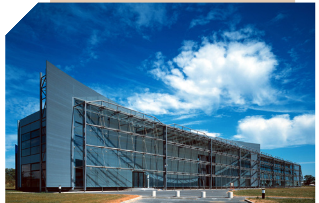
The suspended double glazing façade of the BPO building
